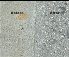
Before and after shot blasting...the profile after should be a little rough. We should discuss with the contractor and make sure that we get the largest machine possible for the project...ask the question as this will impact your schedule if you allow a small machine on site...a small machine is 9"...a good size should just be able to fit through the door.
