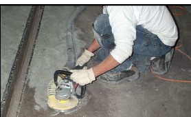
The edges will need to be done with a grinder
